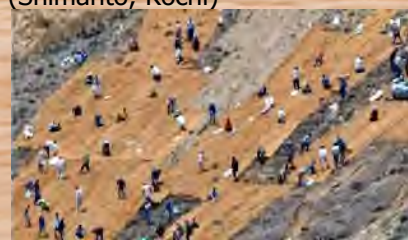
Soil Cover Mats setting to preventing soil erosion (Kami, Kochi)
