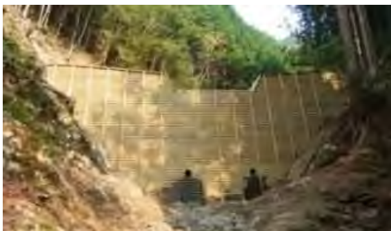
Formwork of dam construction
