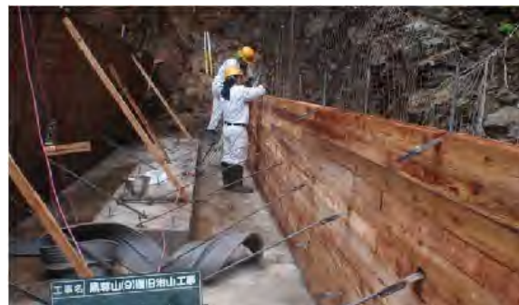
The formwork remains after completion
