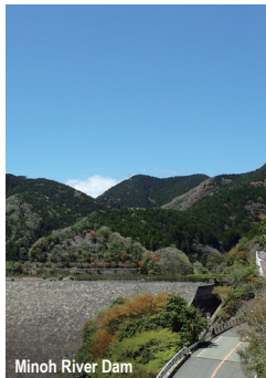
Minoh River Dam
