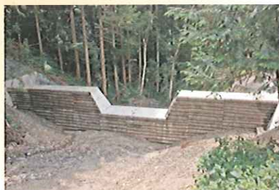
(木製残存型枠工)
