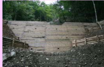
(木製型枠治山えん堤)
