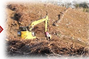
Utilization of grapple machine to the site preparation work
