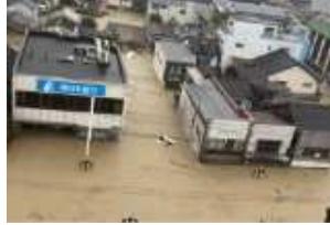
Flooding damage along the Kumagawa River
