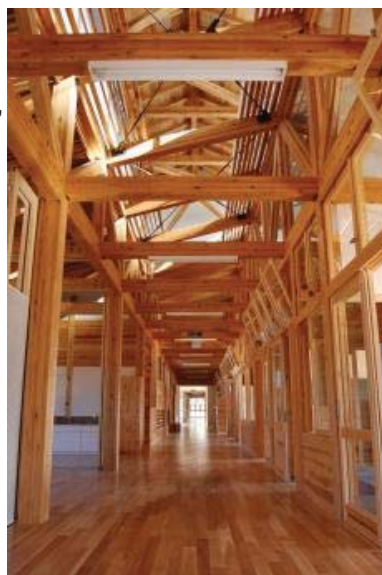
Posts and beams of laminated lumber
