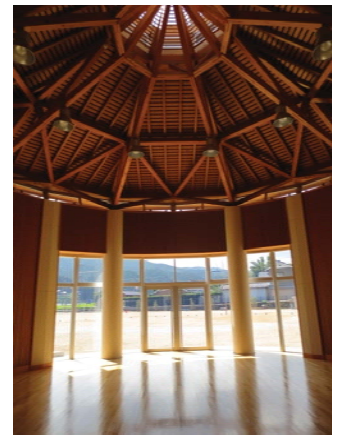
Wood structure of multi-purpose hall
