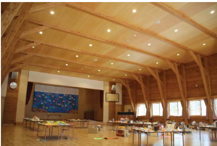
Spacious playroom with two-direction Rahmen (rigid-frame) structure
