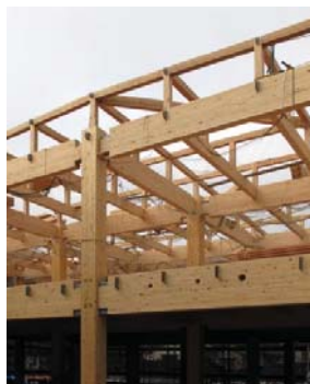
Connecting parts by the LSB system Structural frame in construction
