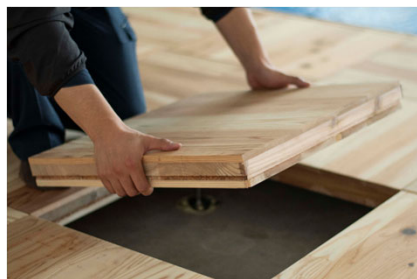
▲WOOD FLOOR UNIT 3.2
