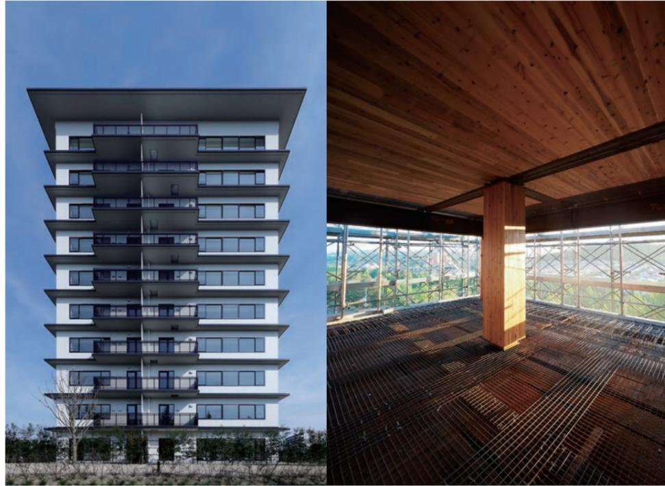
In constructing 10-story apartment building using wood in a portion of the steel frames, technical verification, such as performance of structure, fire resistance and residential quality and shortening construction period, was conducted in this project. In addition, structure lumber which is usually used for low-story building was used. It is expected that such technologies would be applied to non-residential wooden buildings. Such comprehensive approach deserves the Best Award.
