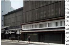
house in Kyoto) built in 1899 and hitherto preserved intact as part of the facility. The common-use area on the irst floor is arranged with traditional building components of Kyo-machiya such as latticework, paper sliding doors and roof trusses in a beautiful and functional manner. Guest rooms are constructed with timber, paper, plaster and other natural materials. Wooden
