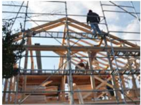
Figure 2-26: Construction Site Assembling Pre-cut Lumber
