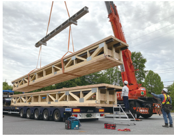
T-WOOD® Truss Floor
