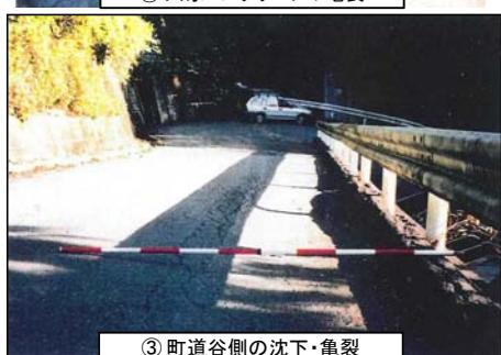
③ 町道谷側の沈下・亀裂
