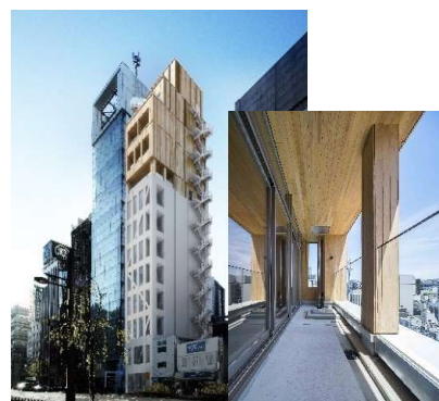
Ginza Takagi Building (Chuo-ku, Tokyo) (©SHELTER CO.,LTD.)
