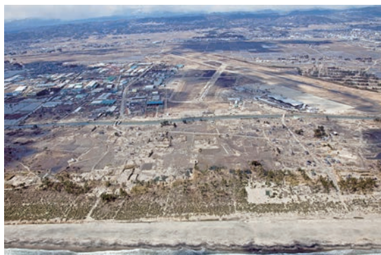
Just after the tsunami (March 2011)
