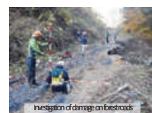
Investigation of damage on forest roads
