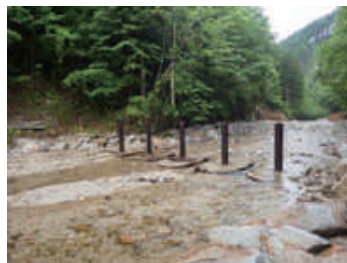
The driftwood catching facility (Tono, District Forest Office) [constructed in 2018]
