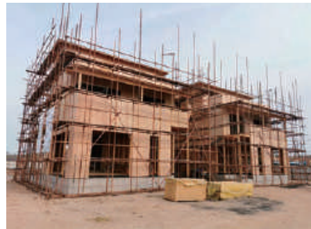
Wood post and beam houses under construction in Dalian, China
