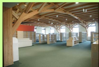
Library built with tree-like braced wooden frame structure (Iwate)
