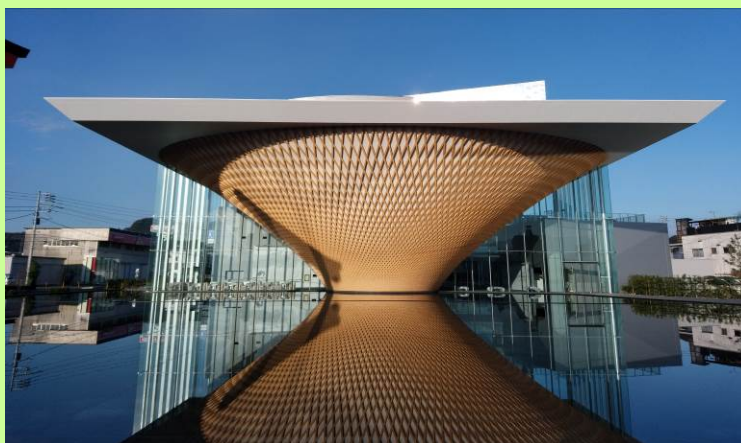
Exhibition facility with wooden lattice using most-advanced pre-cut technologies (Shizuoka)
