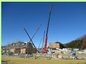
Installation of CLT panels (Fukushima)
