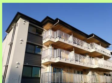
Reconstruction house built with CLT panel structure (Fukushima)
