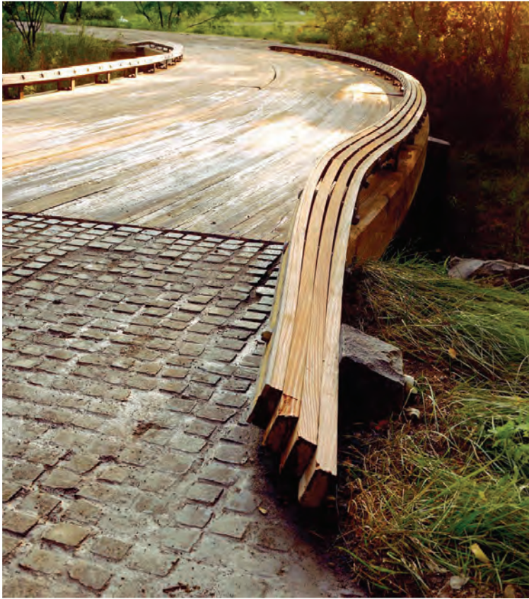
Construction vehicle bridge, curb rail terminus Gray Organschi Architecture/UNALAM
