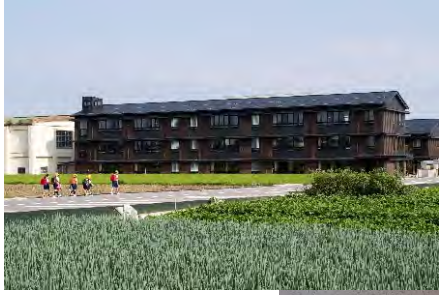
3 story Sawn wood
