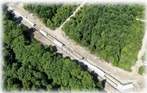
樽前山麓（熊ノ沢）で施工中の導流堤
