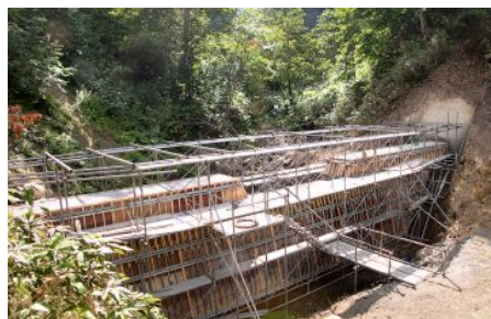
治山工事が進む布引沢
