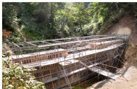
治山工事が進む布引沢
