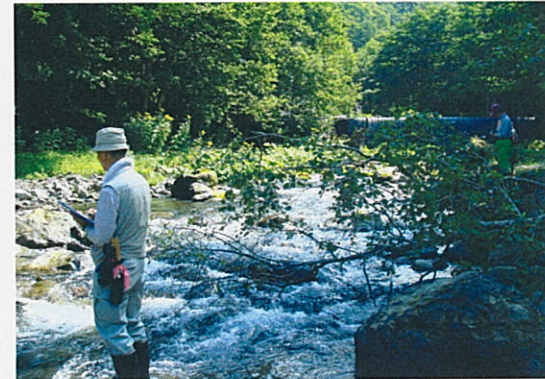
6 Observe further upstream migration of the fish in the upstream of the dam.
