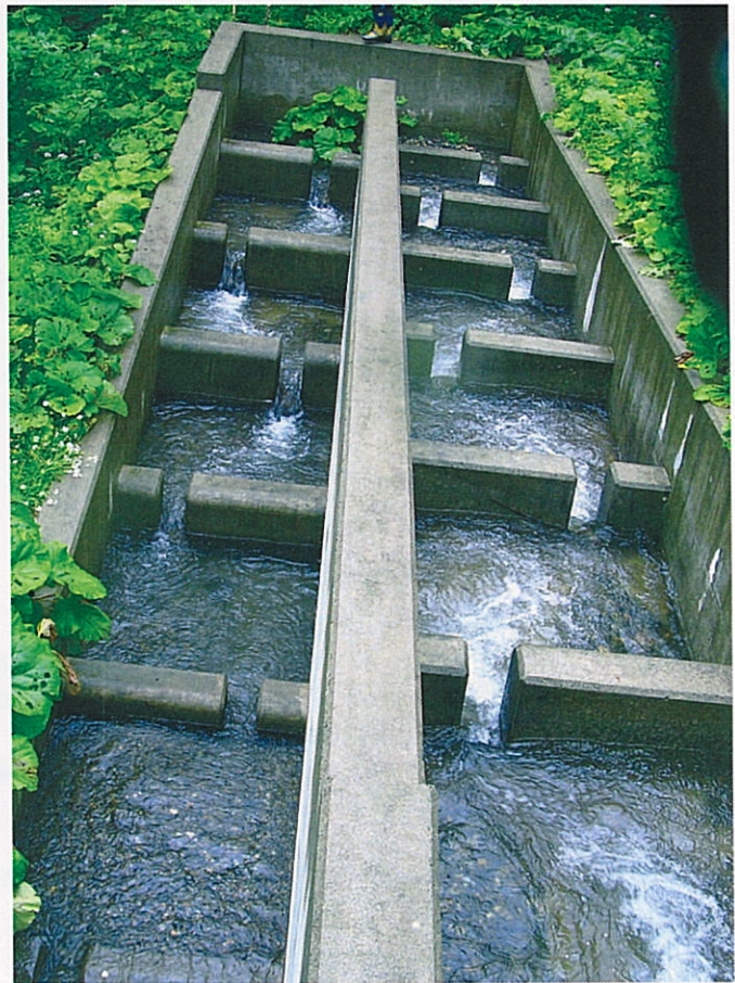
Turn and stair-type Fishway
