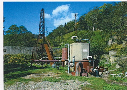
Hot spring facilities under disaster prevention work
