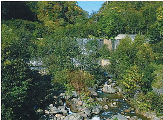
Check dams can prevent sediment disasters and facilitate forest development.
