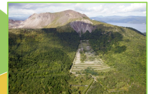
Disaster control facilities of Mt. Usu (Date) [Shiribeshi District Forest Office]
