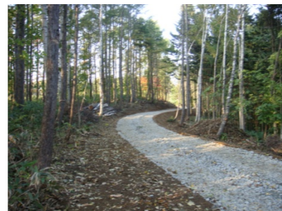
“Forestry exclusive road” for 10-t trucks (National forest in Otaru) [Ishikari District Forest Office]
