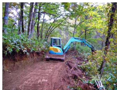
Construction of a “forestry operation road” for forestry machinery such as forwarders (National forest in Shibetsu-shi) [Kamikawa Hokubu District Forest Office]
