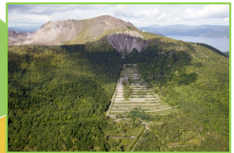
Disaster control facilities of Mt. Usu (Date) [Shiribeshi District Forest Office]
