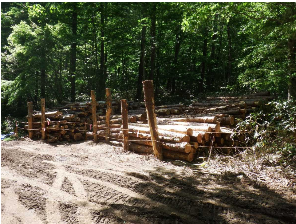
森姫川治山工事支障木
