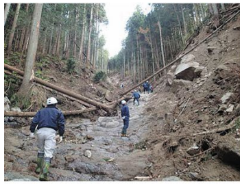
East Japan typhoon in 2019 Marumori-Town, Miyagi Prefecture (Longitudinal erosion of mountain streams: 2-3m)
