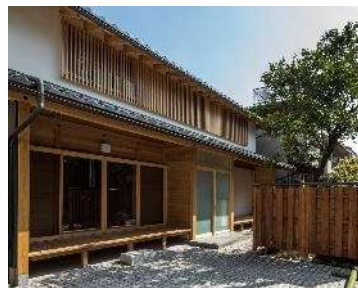
Fireproof construction using thick cedar boards to realize exposed wood exterior
