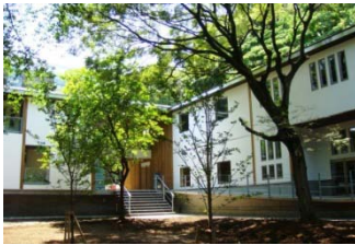
Photo: Education and research support facility in the University of Tokyo. Built with generic lumber with post-beam structure.
