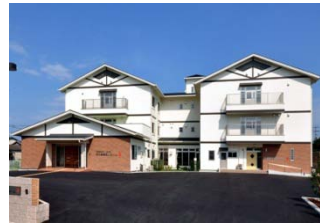
Photo: Special facility for the elderly in Tamano, Okayama Prefecture. One of the largest fire-resistant wooden buildings in Japan.
