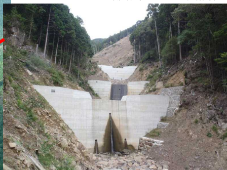
(溪間工施工箇所)
