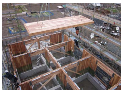
Apartment building being constructed using CLT (Maniwa City, Okayama Prefecture)
