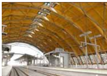
Kochi Station: A Station Built with Regional Wood (Kochi City, Kochi Prefecture)
