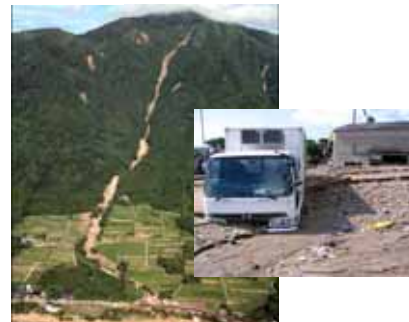
Damage from Typhoon #4 (Minami-Osumi Town, Kagoshima Prefecture)
