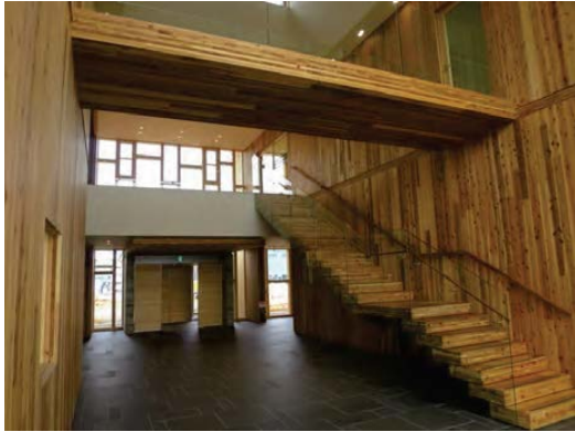
Photo ii: Building using CLT (Kochi prefecture)
